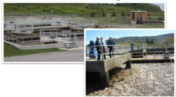
Conventional Activated Sludge Treatment
