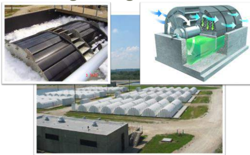
Rotating Biological Contactor
